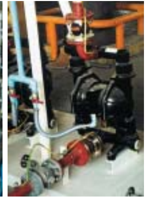
ARO diaphragm pumps used in chemical laboratory.
