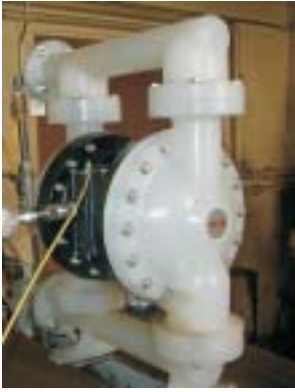
EXP pump has replaced competitive model to reduce air consumption
